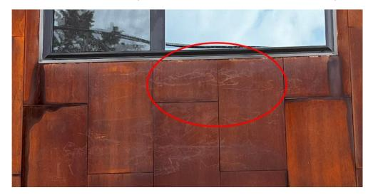
Also, you can see that he accelerator that was used has not been fully removed and neutralised and is leaching out from the gaps in the panels and window frames (Dark Wet areas). This has caused the surface to flake and over time may cause more serious damage within the panel gaps.
